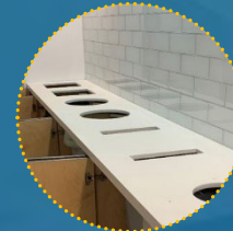
Countertop cut-outs for touchless waste and recycling system
