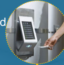
Touchless destination dispatch system via card or mobile app. Keep elevator doors open at lobby/floors (note stack effect concern in winter)
